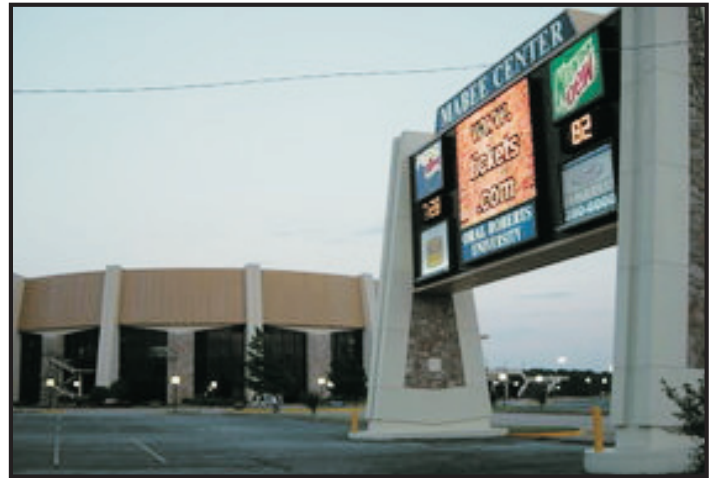
The Ecoglo installation at the Mabee Center was more complicated than for standard arenas because of the center's cambered and fully carpeted steps.
