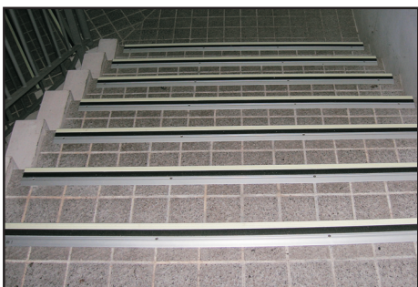
Step nosing can be installed easily onto substrates such as concrete, tile, wood, carpet, vinyl, steel and aluminium
