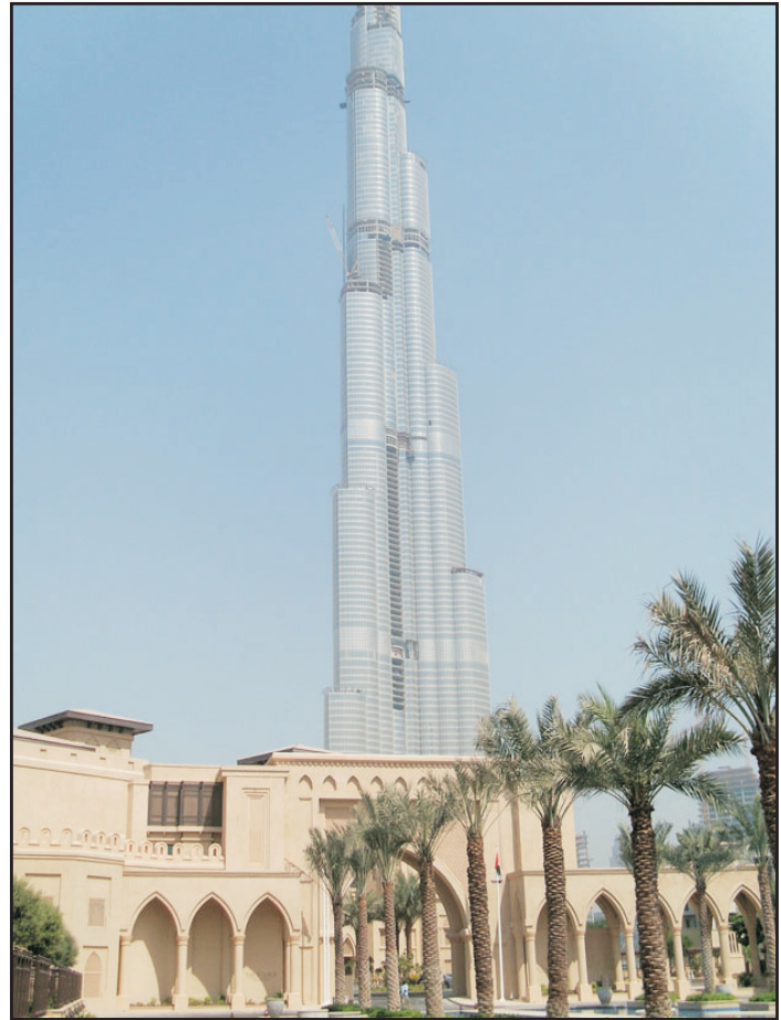
The 160 storey multipurpose Burj Dubai, already dwarfing its neighbours, is due for completion in September 2009.
